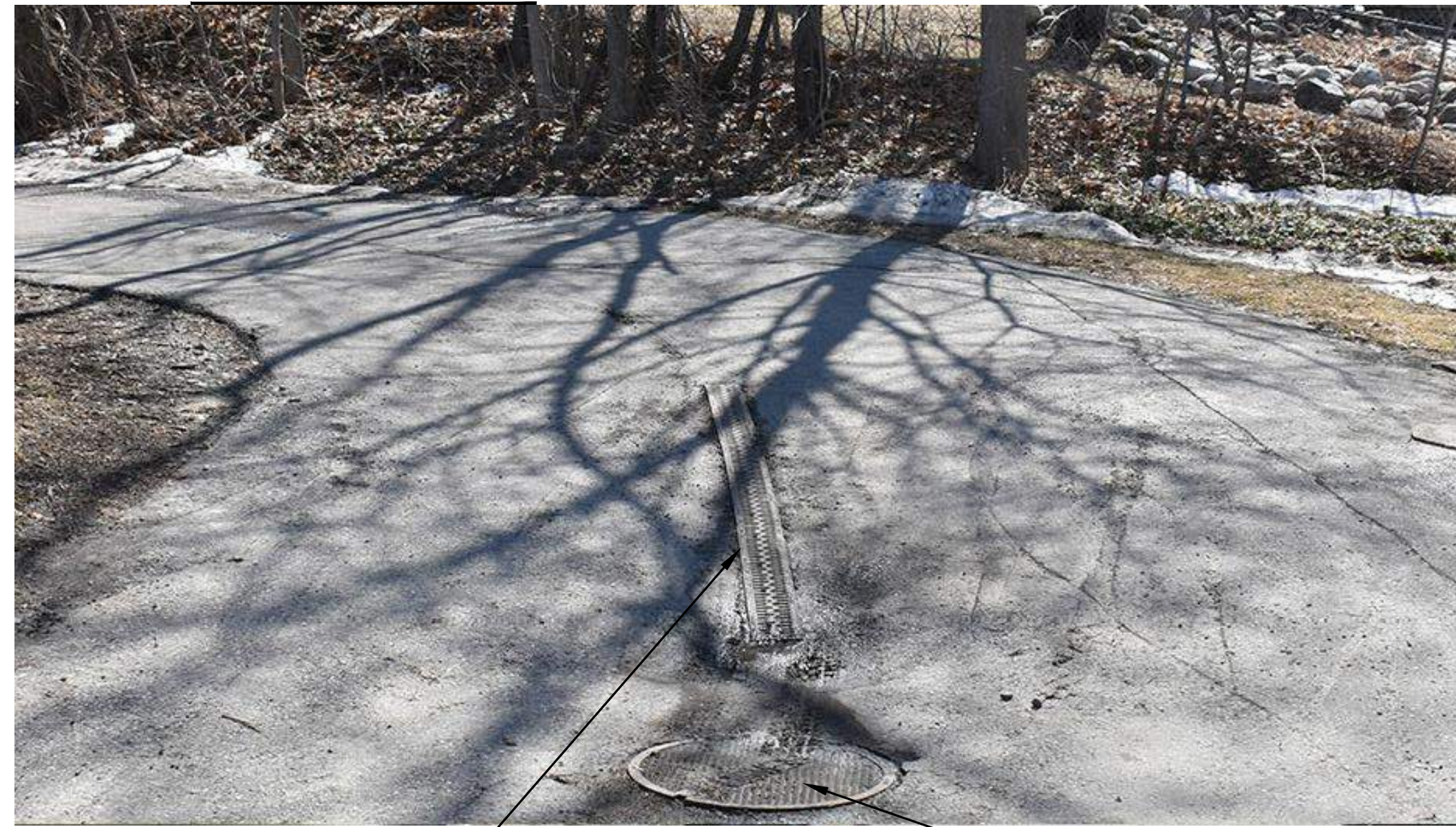
WASH WASTE WATER COLLECTION GRATE
